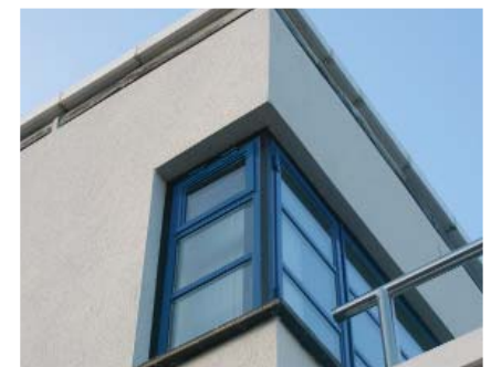
Corner Superlintels with Duragalv 140 met 90 years component service life demands at Lynton Lifeboat station, near Southampton.
