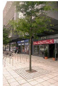
Photo ref: Bristol 5075 Softening urban landscaping with tree planting – recessed tree grids allow maximum paviour coverage, reducing the risks of slips and trips and easing passage across for wheelchairs in response to the DDA.
